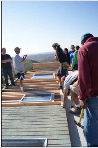
Building the first wall
