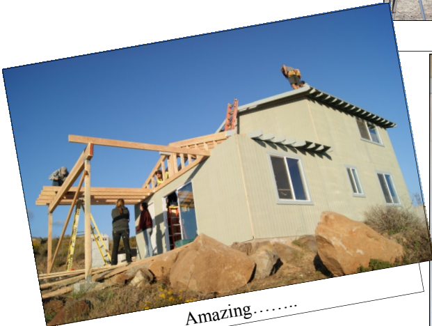
Framing the upper floor
