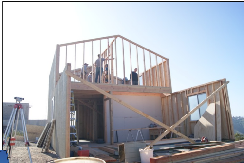
Framing the upper floor
